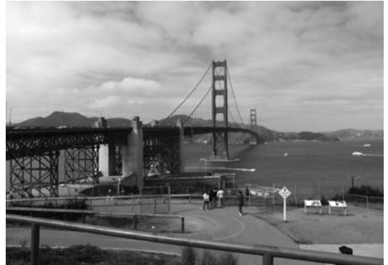
Golden Gate Bridge
